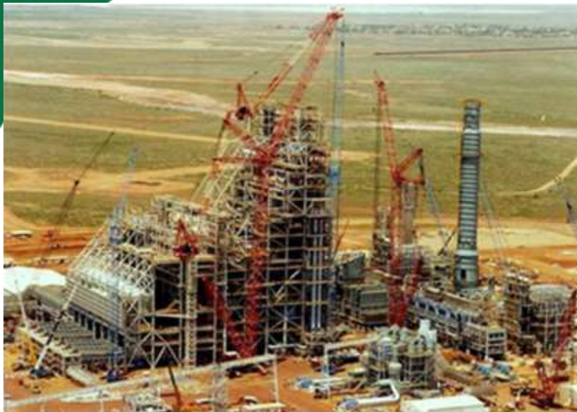
BHP HBI Project During Construction
