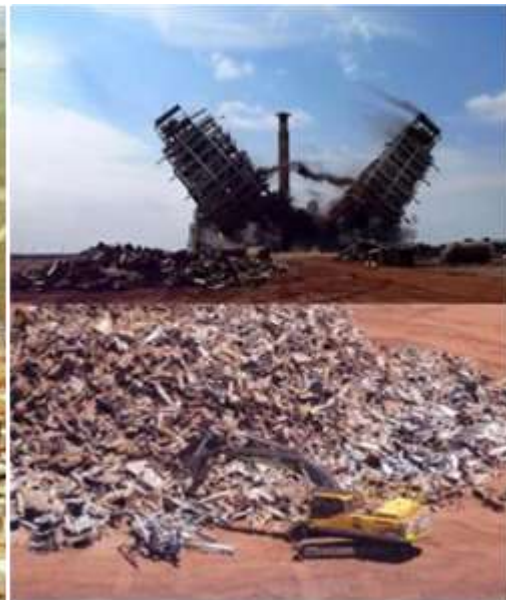
Plant was shut down then razed to the ground
